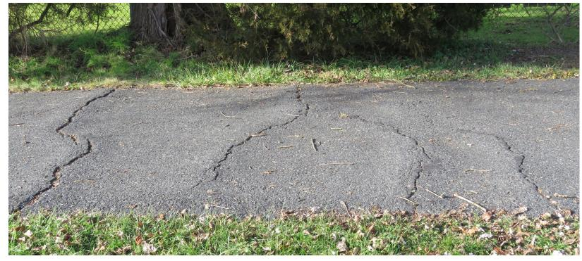
Walking path is badly buckled in many areas, presenting trip hazards and making alternative uses such as roller blading impossible
